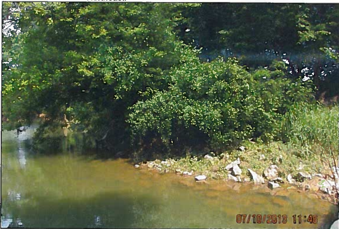
Photograph No. 4: View of North Embankment Downstream of the Structure, Looking Northwest.
