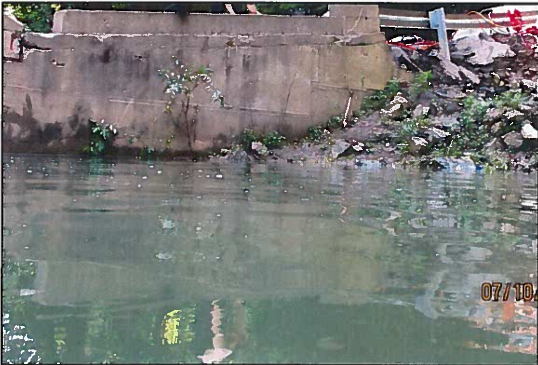
Photograph No. 9: View of West Wingwall of Abutment 1, Looking Southeast.
