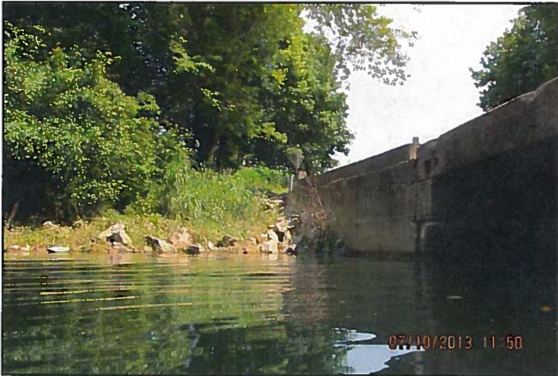
Photograph No. 13: View of West Wingwall of Abutment 2, Looking Northeast.
