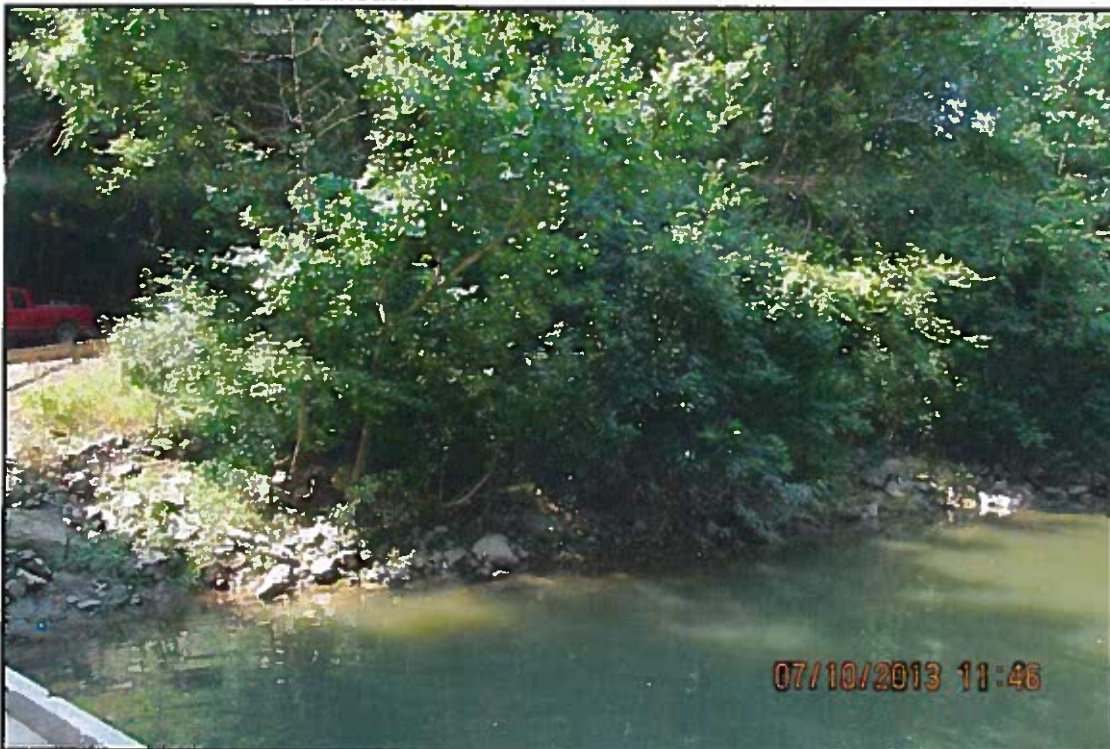
Photograph No. 6: View of South Embankment Downstream of the Structure, Looking Southwest.
