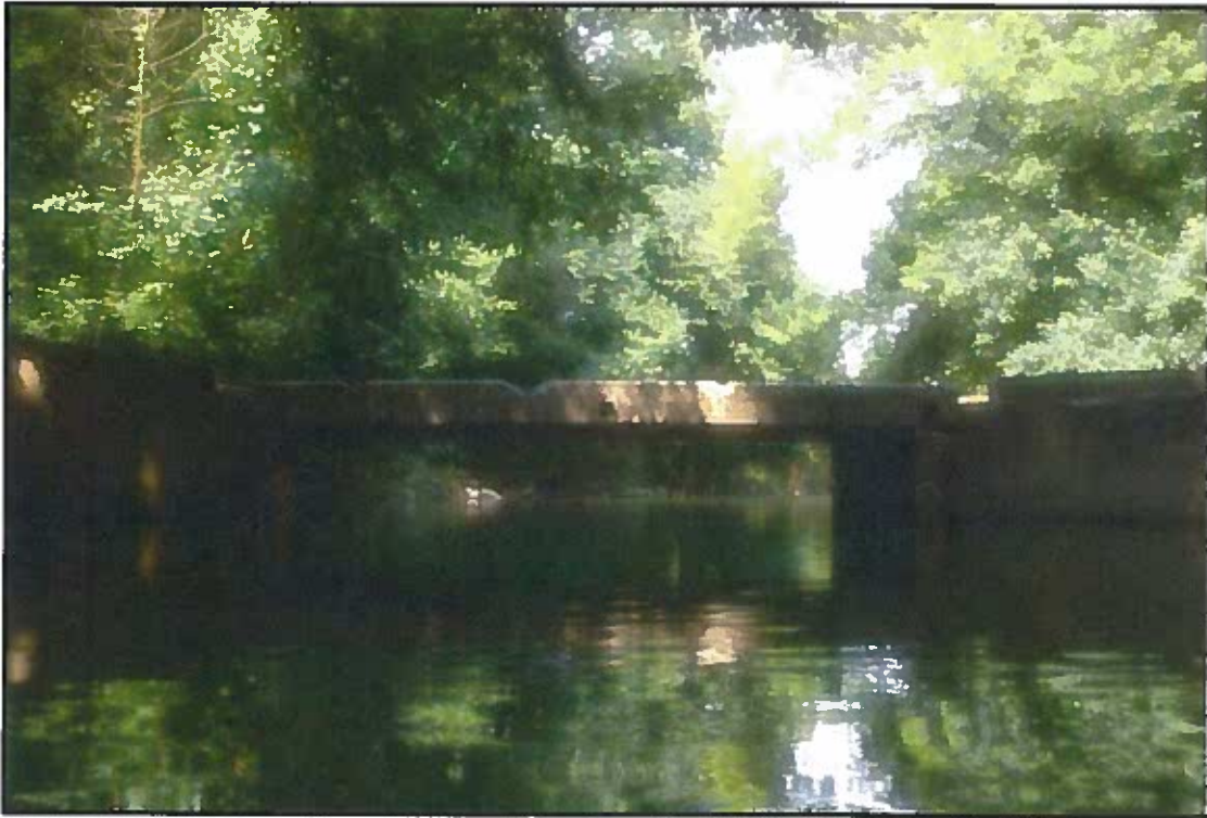
Photograph No. 1: Overall View of Structure No. 108B00041N, Looking West.
