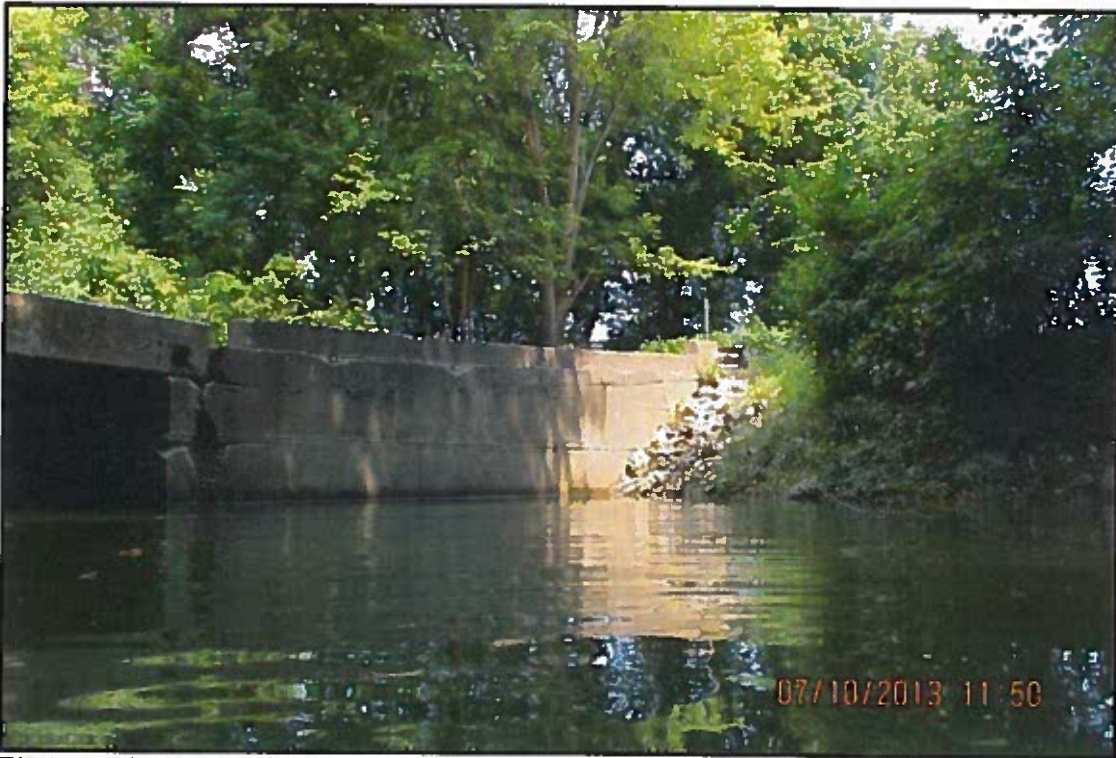
Photograph No. 11: View of East Wingwall of Abutment 2, Looking Northwest.
