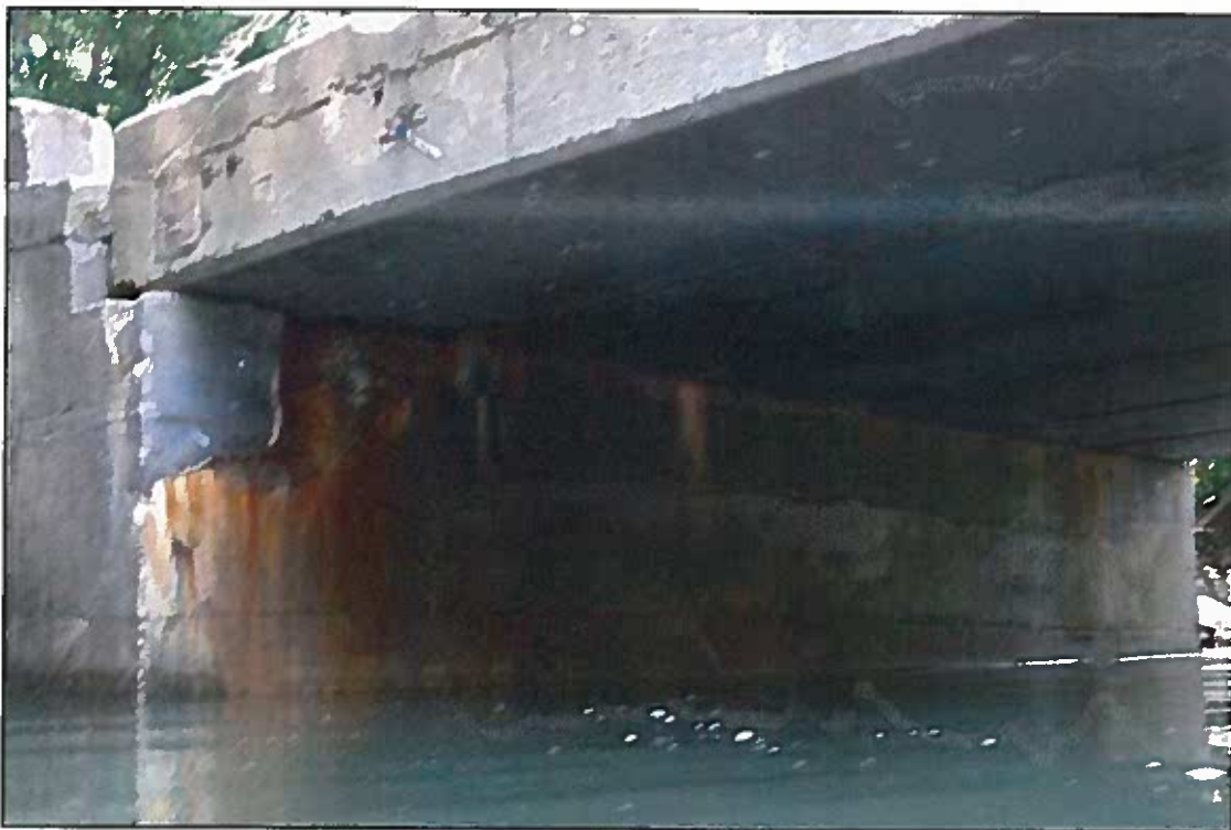
Photograph No. 8: View of Abutment 1, Looking Southwest.
