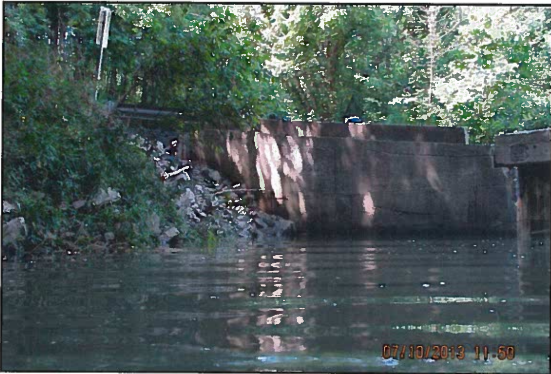
Photograph No. 7: View of East Wingwall of Abutment 1, Looking Southwest.
