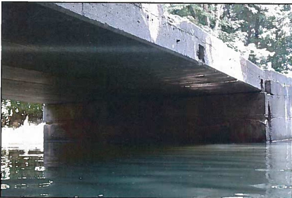
Photograph No. 12: View of Abutment 2, Looking Northwest.
