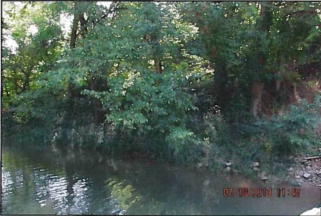
Photograph No. 5: View of South Embankment Upstream of the Structure, Looking Southeast.
